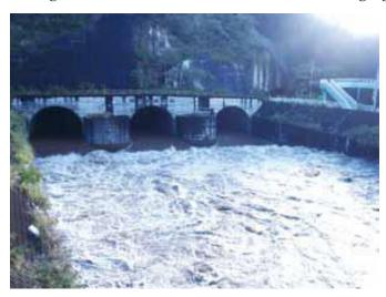
In heavy rain or typhoons the gate of movable dam is opened and can discharge the water of the maximum 2,000 m<sup>2</sup>/second.
